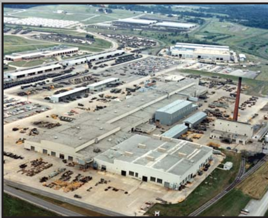
An ariel view of the completed buildings 350, 370 and 320 ready for the new Paladin mission as well as other tracked, wheeled vehicle projects and the new missile workload.
